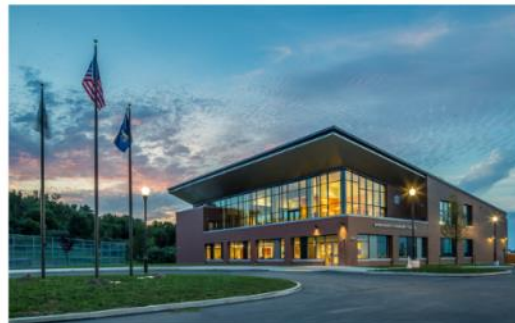
North Fayette Township Community Center
